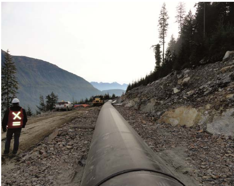
Box Canyon Hydro - Penstock
