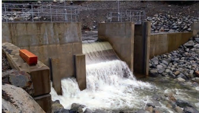
Right: Marty Creek main intake, showing Coanda screen and maximum diversion control weirs.
