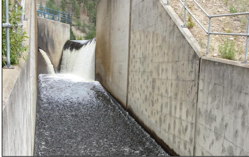
Figure 4: Spillway Outlet Channel
