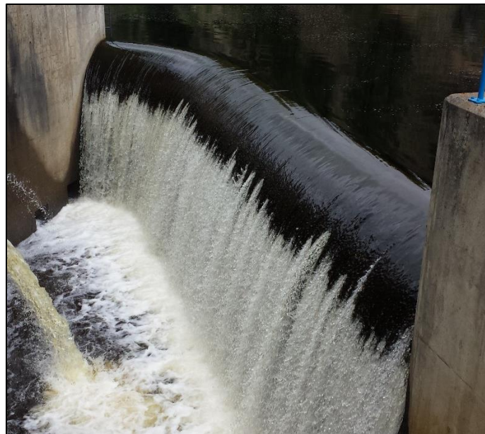
Figure 3: Spillway Overflow Weir
