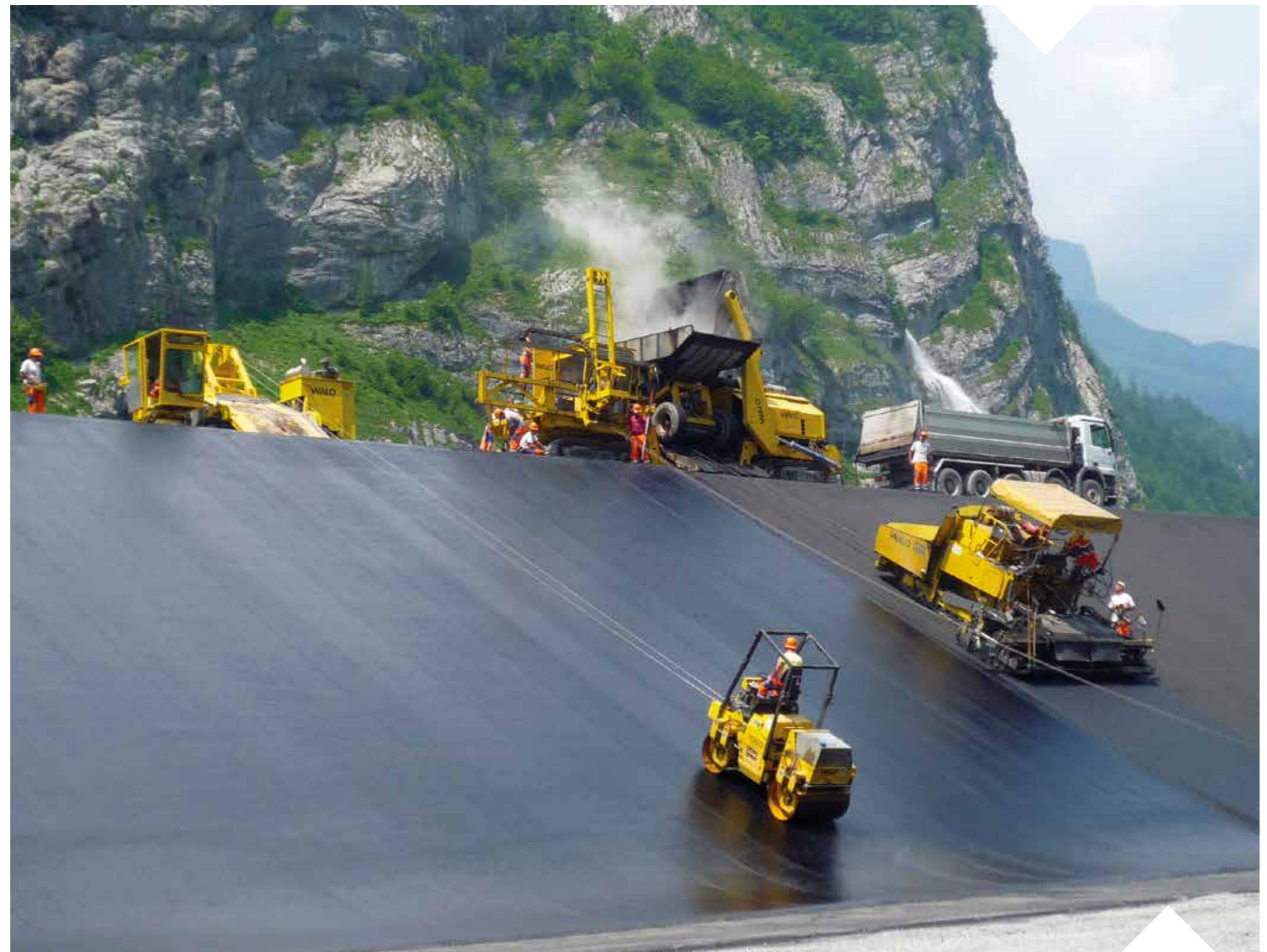
(Above) Example of placing and compacting a new dense asphalt concrete, done on a dam similar to the Von Bach Dam.
