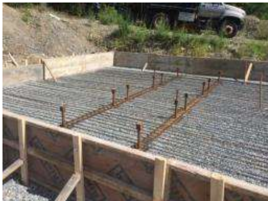
Photo 4 - Welded embedments for anchoring structure to base slab
