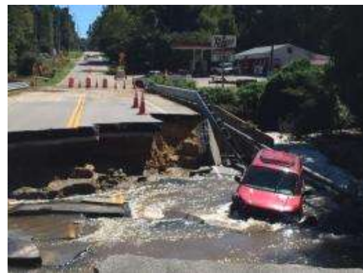
Photo 1 - Lake Elizabeth Dam Failure, SC (October 7, 2015, credit: Jacob Haskew, WBIR News)
