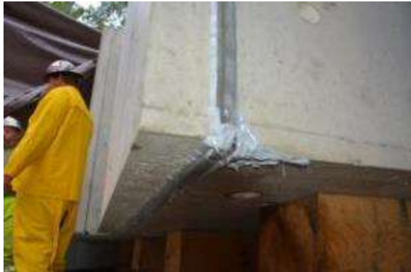
Photo 6 - Expansive waterstops used to seal joints
