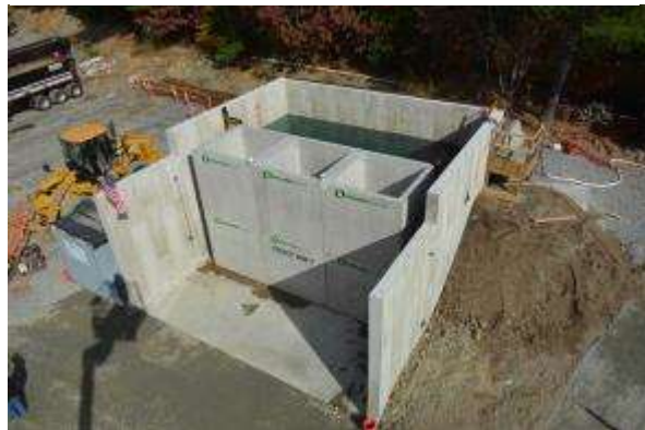
Photo 9 - Fully-assembled dam with full reservoir
