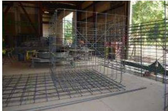
Photo 3 - Reinforcement cage for upper-tier module
