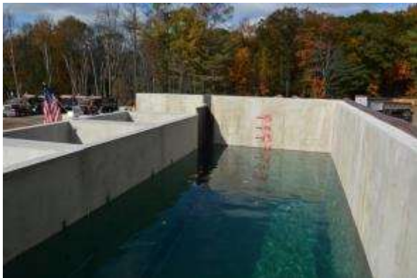
Photo 8 - Tank filled with approximately 30,000 gal of water for up to 12 ft head
