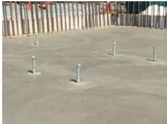
Photo 5 - Bolts installed in couplings prior to concrete placement
