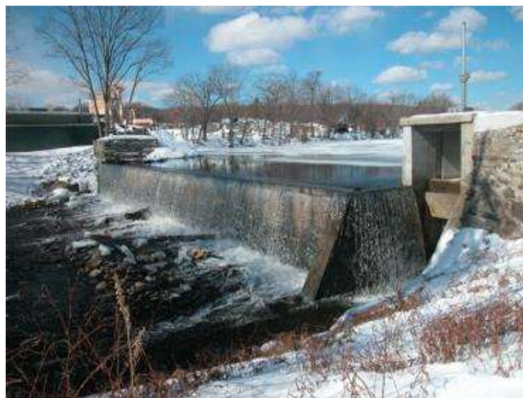
Photo 10 - Unnamed CIP dam, Rhode Island
