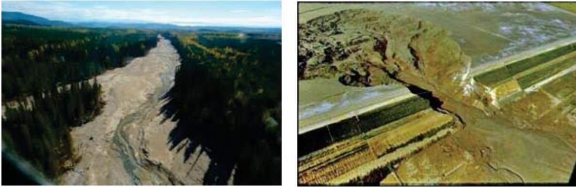
Figure 1. (a) Erosion caused by the initial flood wave following the Mount Polley dam failure (MPMC, 2015); and (b) Cone of depression of slumped liquefied tailings caused by the Merriespruit dam failure (www.tailingsinfo.com, 2015)
