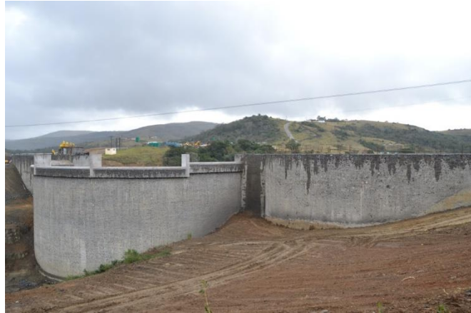
Figure 8. Mndwaka Dam – view from upstream face
