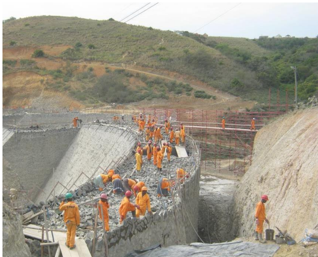
Figure 7. Mndwaka Dam – construction
