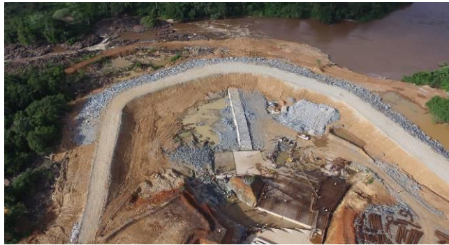
Figure 12. Azambi HPP – stage 1 diversion works
