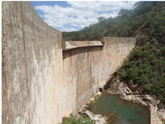
Figure 2. Lucilia Poort Dam Wall – RMC arch structure
