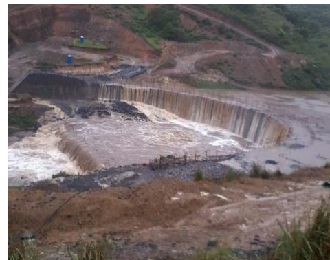
Figure 5. Mndwaka Dam – central arch overtopping during construction
