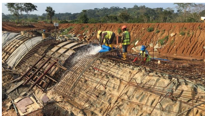
Figure 11. Azambi HPP – construction of spillway crest cap
