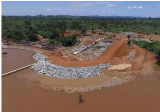
Figure 13. Azambi HPP – stage 2 diversion works
