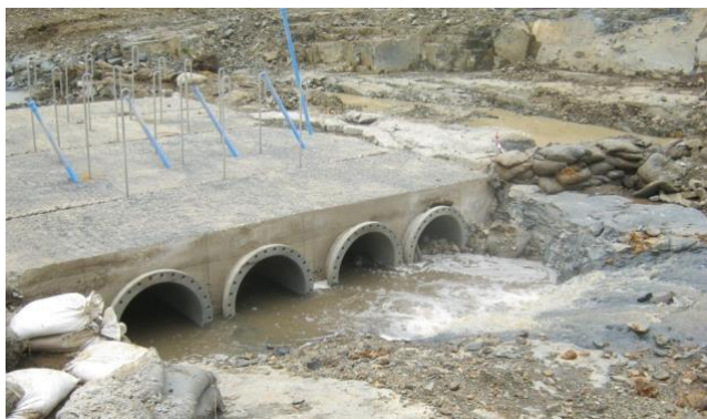
Figure 4. Mndwaka Dam – river diversion structure
