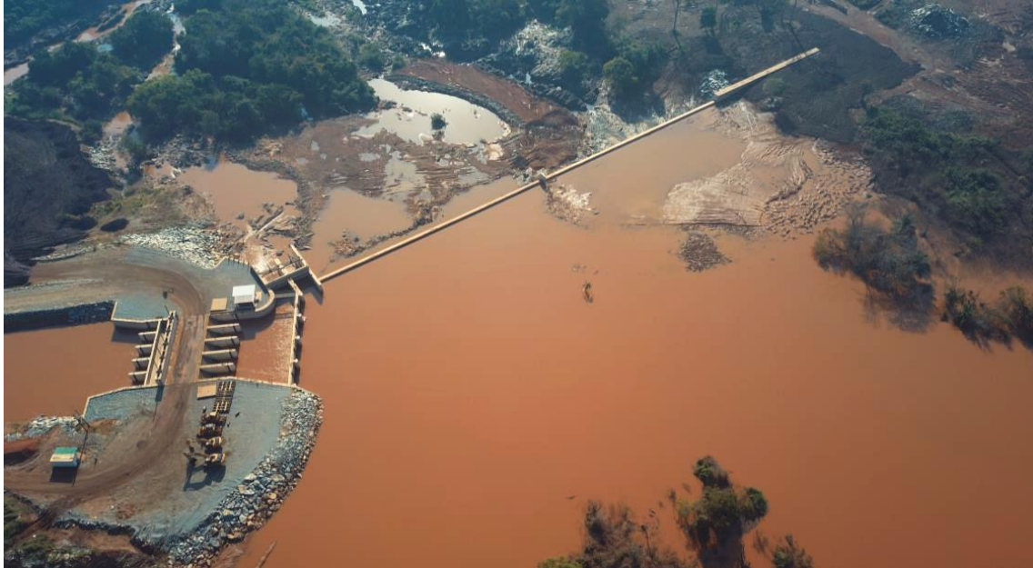
Figure 14. Azambi HPP – completion of RMC diversion weir
