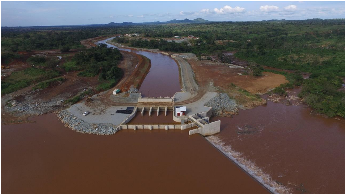
Figure 9. Azambi HEP – RMC diversion weir, intake structure and power canal
