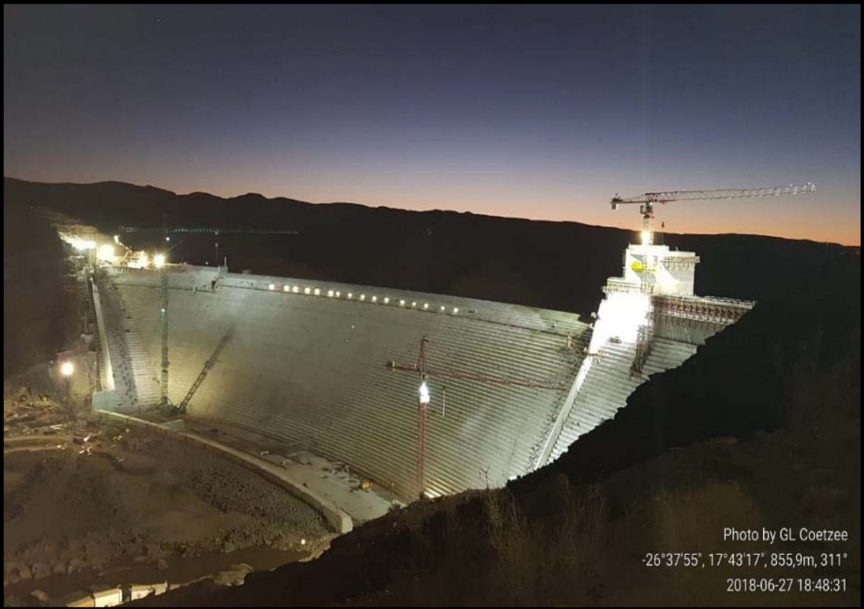
Figure 1: Neckartal Dam June 2018 (View from downstream - top of the left bank)
