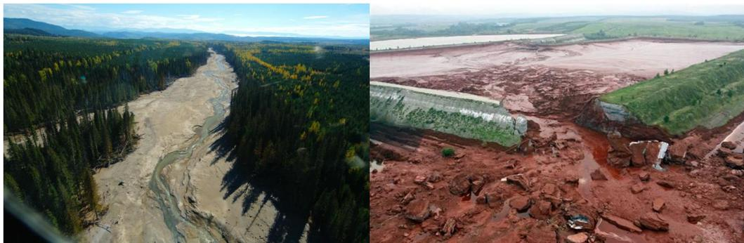
Figure 1: (a) Erosion caused by the initial flood wave following the Mount Polley dam failure (MPMC, 2015); and (b) Cone of depression of slumped liquefied tailings caused by the Kolontár dam failure (Oszvald, 2015)
