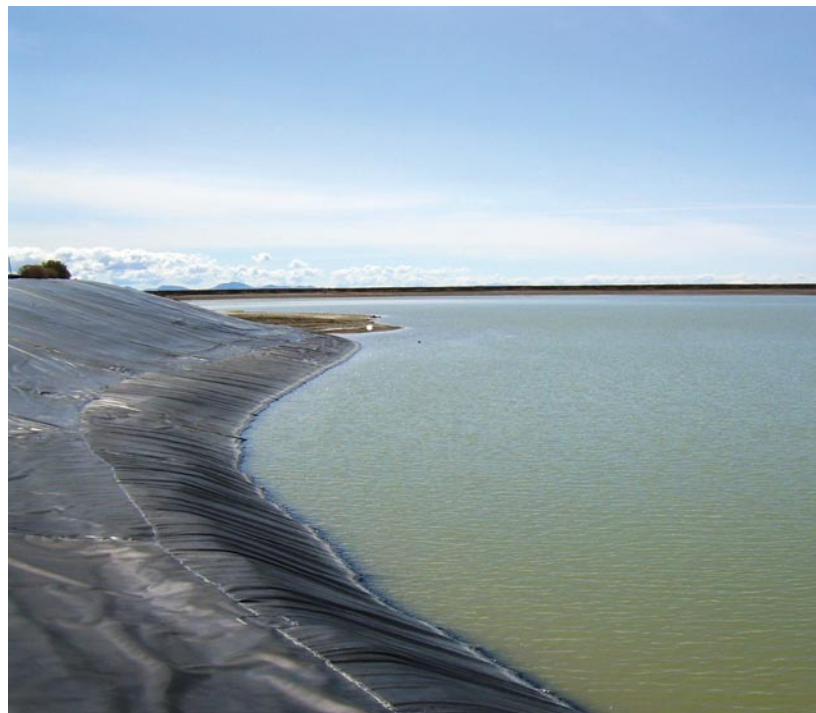
A geomembrane lined tailings facility.
