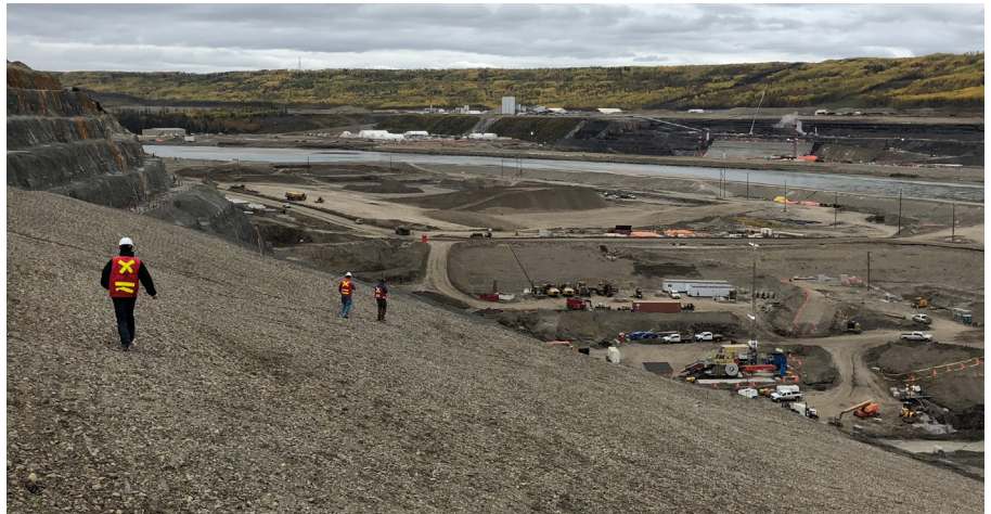
Six large cofferdams diverted the Peace River and enabled the construction of the permanent works.
