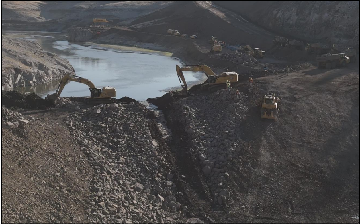
Figure 6: Breach Initiation with Long Arm Excavators
