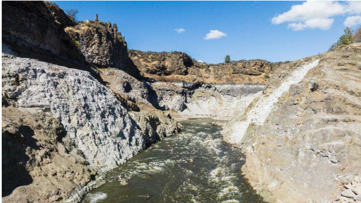
Figure 4: Klamath River channel at the former Copco No. 1 Dam site, looking upstream. (Credit: Kiewit)
