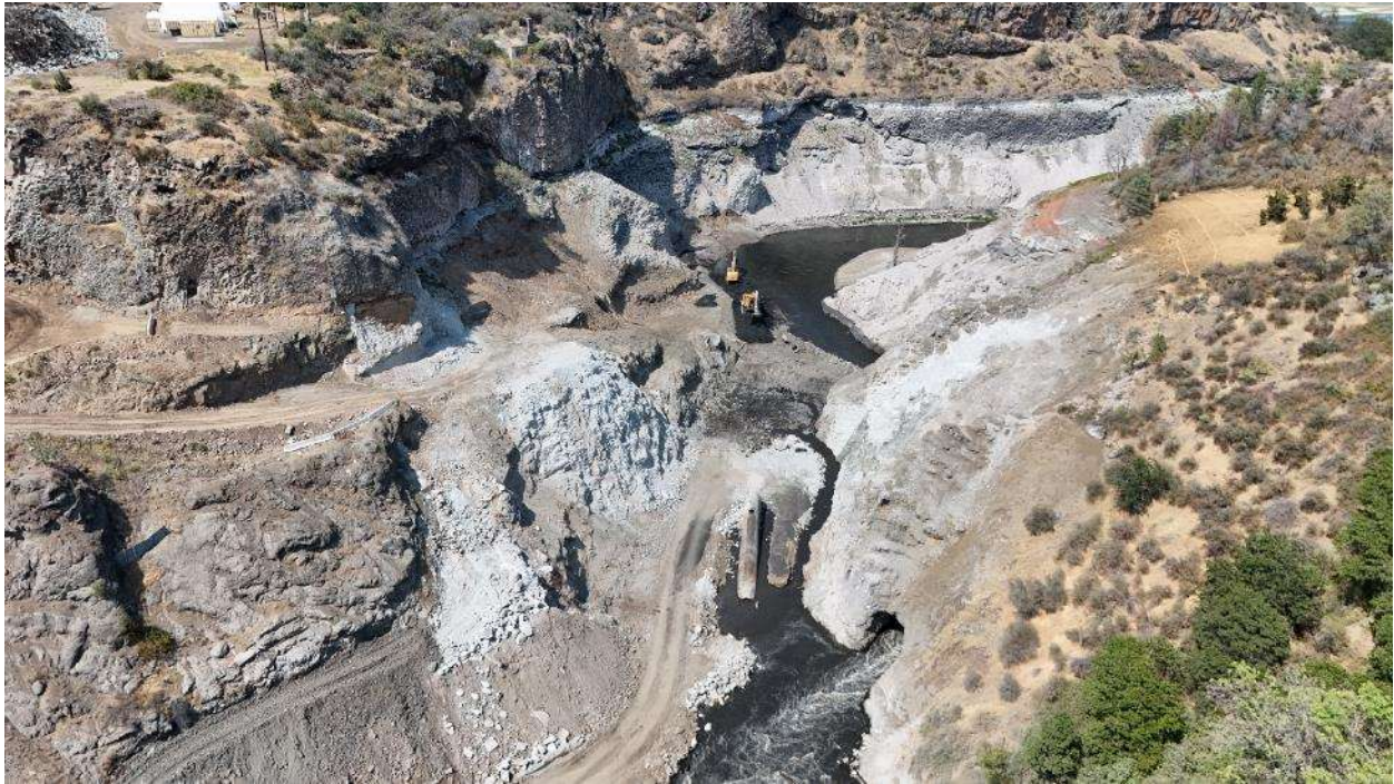
Figure 3: Concrete excavation for dam removal. Klamath River is diverted through the diversion tunnel. (Credit: Kiewit)
