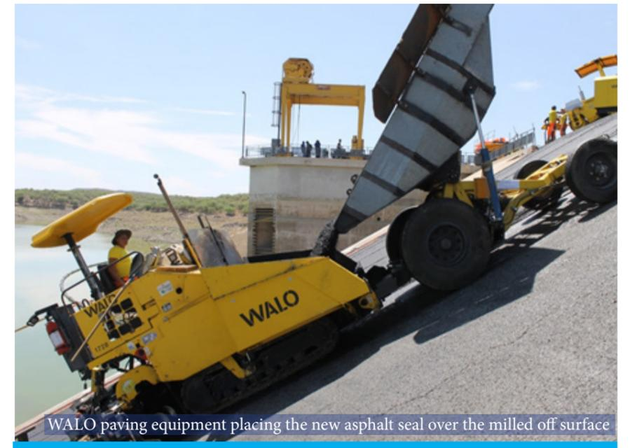
WALO paving equipment placing the new asphalt seal over the milled off surface
