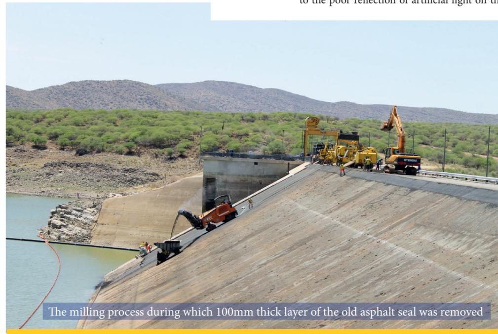
The milling process during which 100mm thick layer of the old asphalt seal was removed
