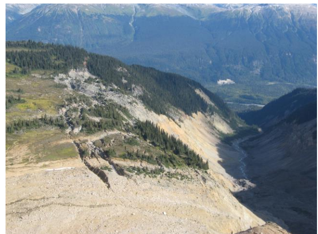
Photo 1. Sacking features with extensive tension cracks in the Affliction Creek Catchment.
