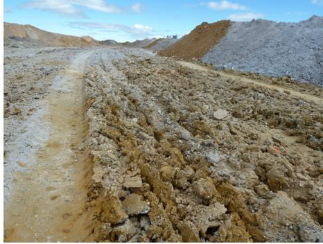
**Figure 7: Scarification between layers**
