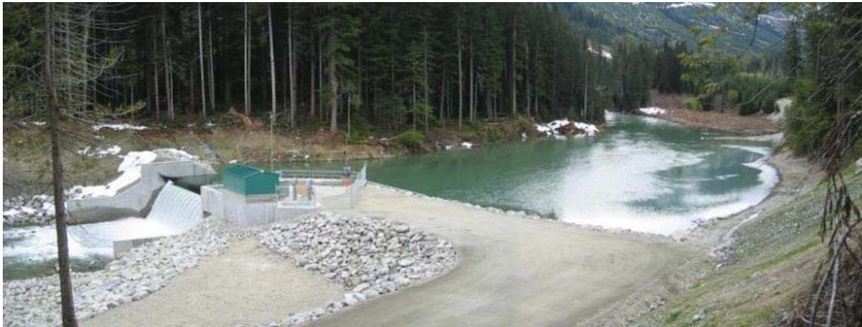
**Figure 2. Rutherford Creek 49 MW Hydro Project - Inflatable Rubber Dam**
