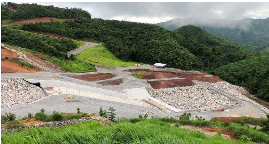
Figure 1. Phu Kham Emergency Spillway – Photo of Stage 2 spillway raise
