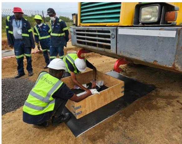
Fig. 4. Testpad under construction to monitor damage and strain in the geomembrane.
