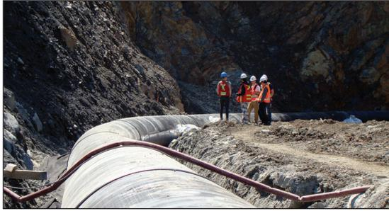
Nine intake structures feed into this high-pressure penstock.
