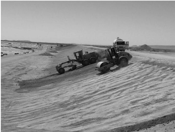
Figure 5. TSF Starter wall compaction
