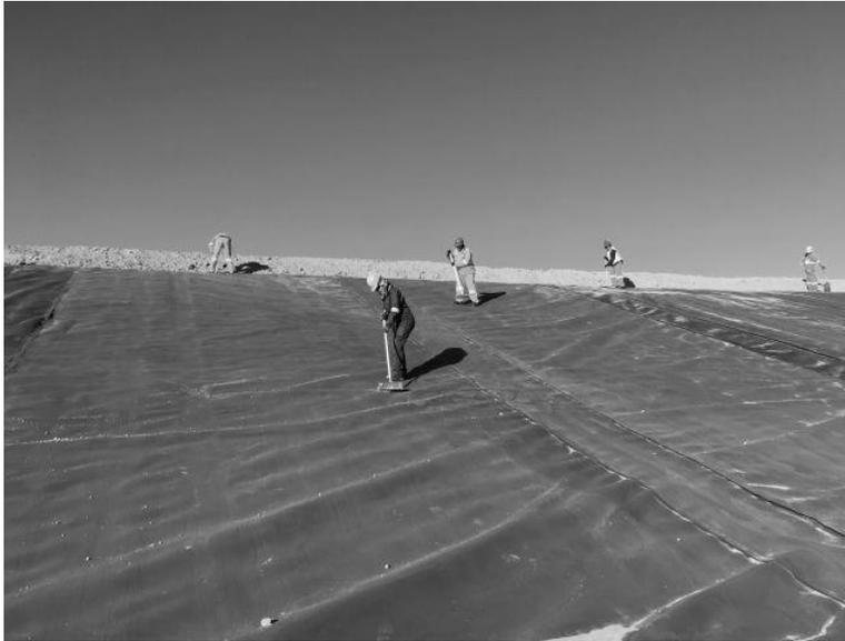
Figure 6. TSF Starter wall cleaning
