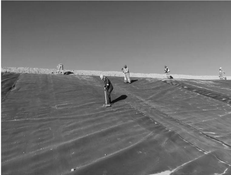
Figure 6. TSF Starter wall cleaning
