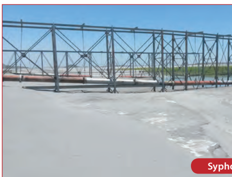
Lining of TSF's
