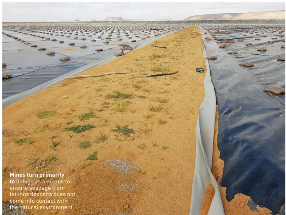
Mines turn primarily to linings as a means to ensure seepage from tailings deposits does not come into contact with the natural environment
