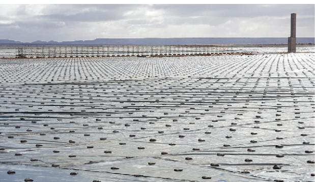
or a more natural substance such as clay which can be costly to use if it does not occur naturally on site, influences the design of the facility and more importantly, the stability of the structure. A layer between the ground and a large mass of loose/unconsolidated material weakens the facility, in most cases.”
