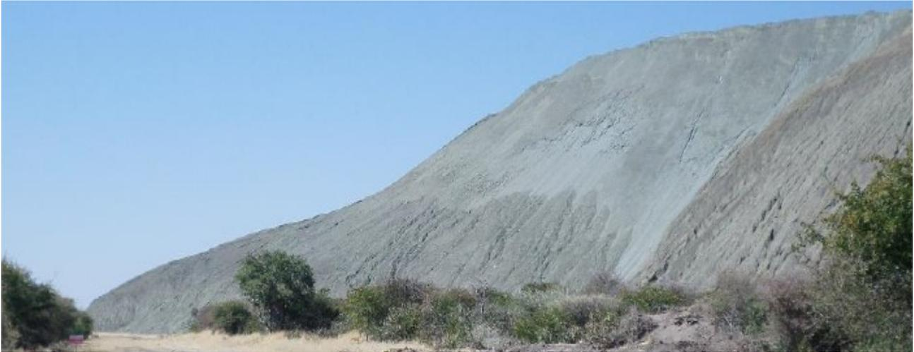
Figure 3 Photograph of a tailings dump that has slumped (bulge and nose)
