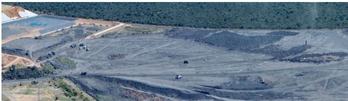
Figure 12 Load and haul dry ash operation using trucks and bulldozers
