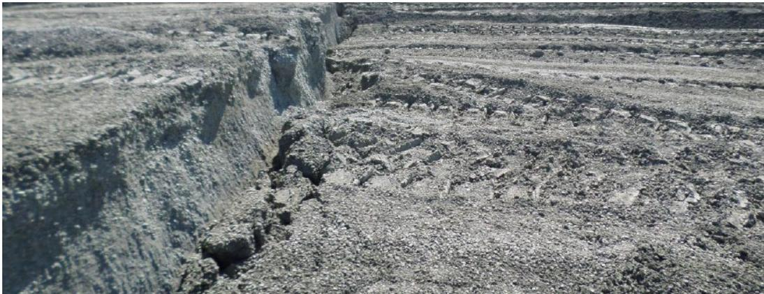
Figure 9 Photograph of a dump that has settled (failed) – tension crack formed
