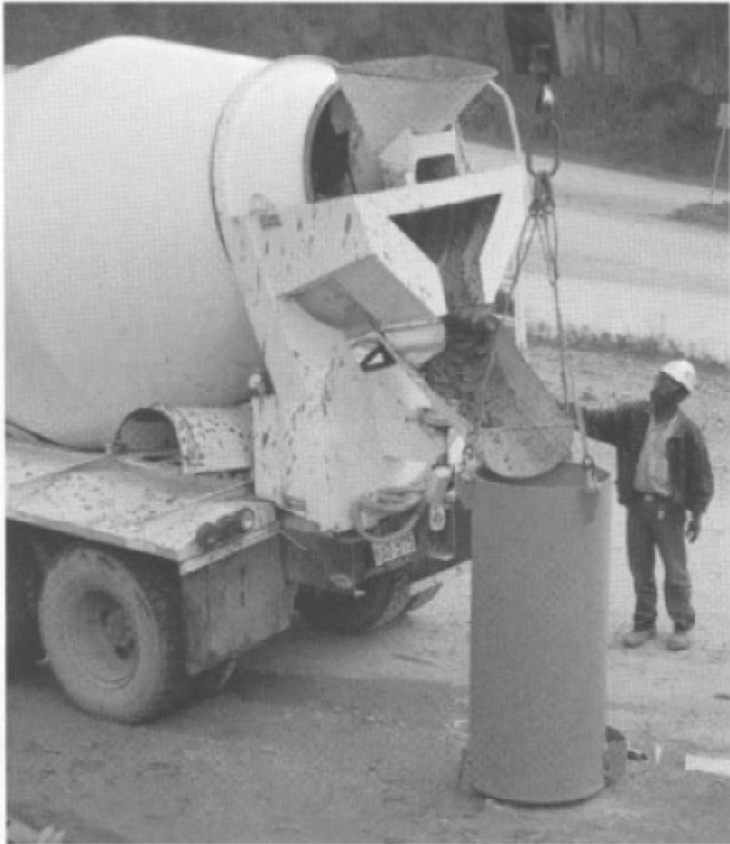
*Figure 2 Concrete transit mixer truck and skip*
