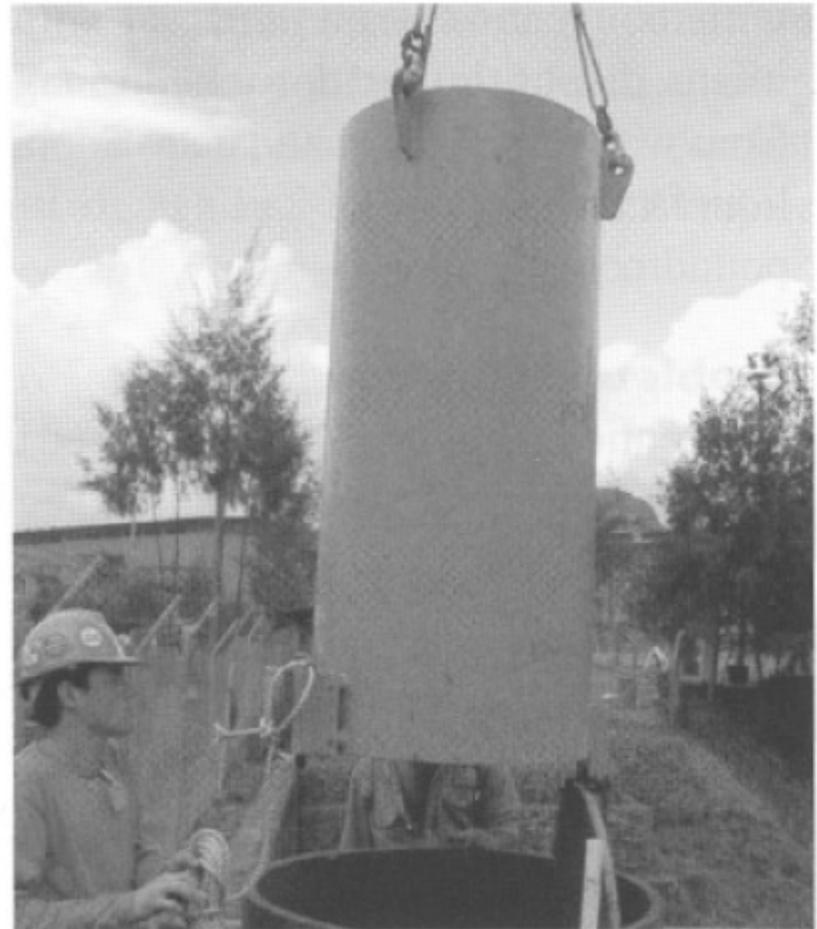
*Figure 3. Skip during column loading*
