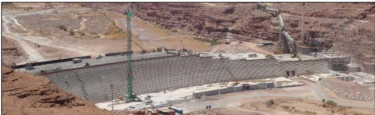
**Figure 2. RCC on 7 steps during the construction of the dam wall**
