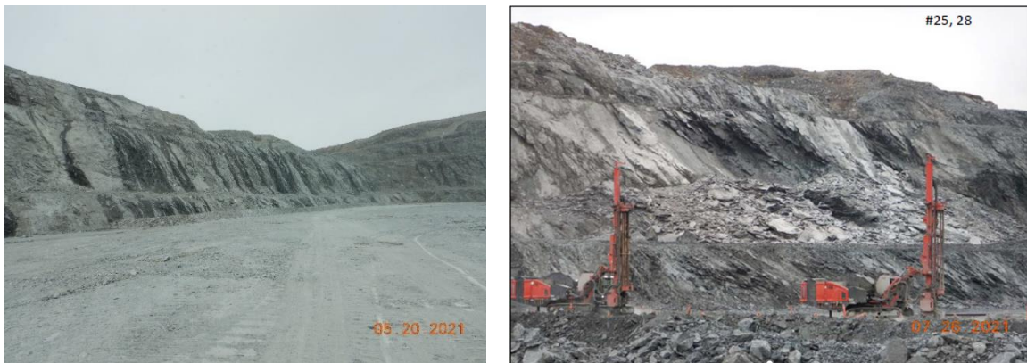
Figure 10 : 2021 – Phase 3 Northwest Wall Before Freshet (Left) & During Freshet (Right)
