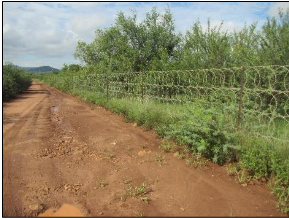
Plate 1 :Gravel access road and razor-wire boundary fence
